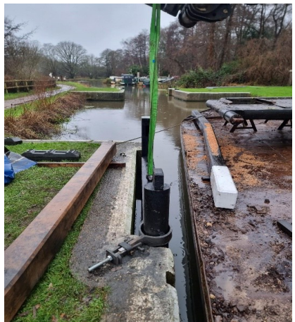
Walsham Flood Gates Replaced
