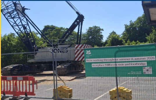
Site Set Up for Millbrook Weir Rebuild
